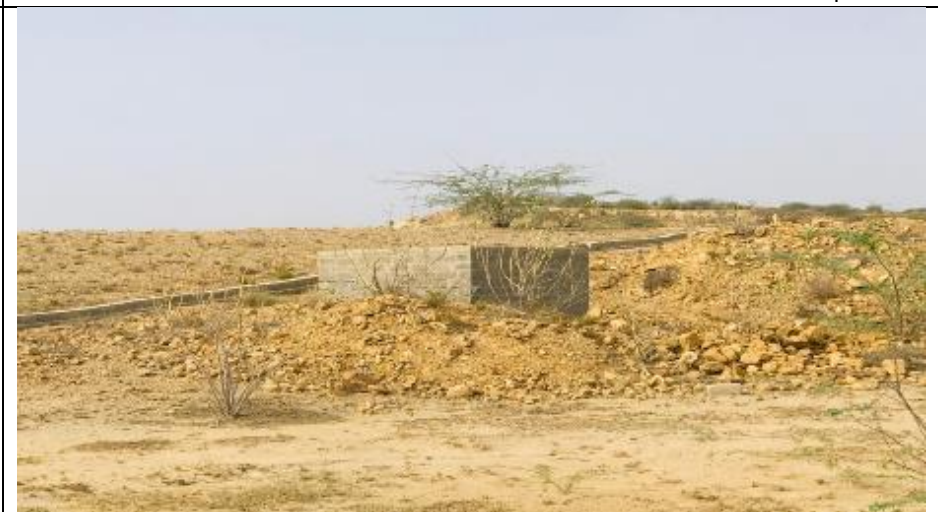
01/07/24 – Deh Halkani & Deh Bund Murad – Abandoned Structure
