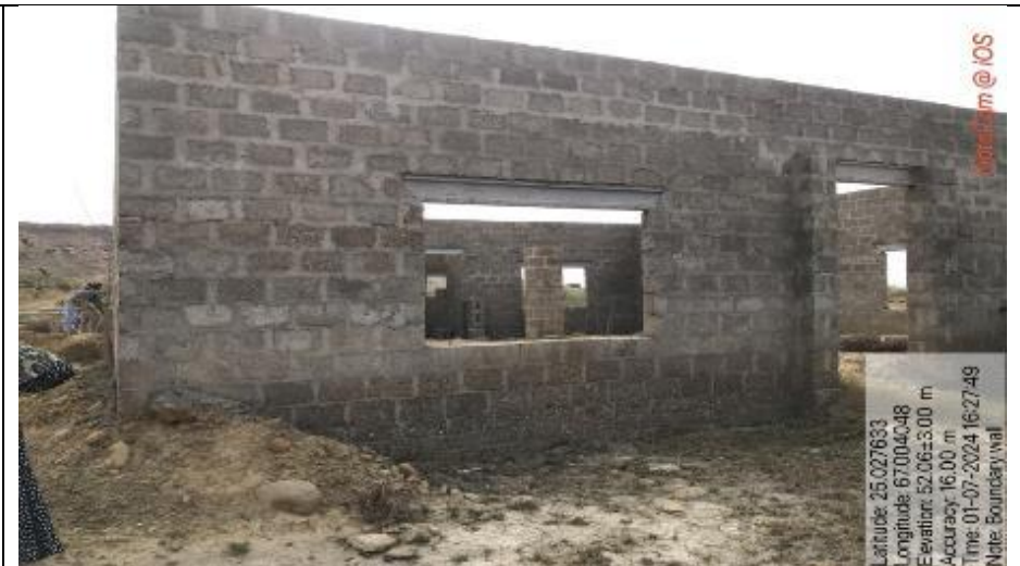
01/07/24 – Deh Halkani & Deh Bund Murad – Under Construction Mosque
